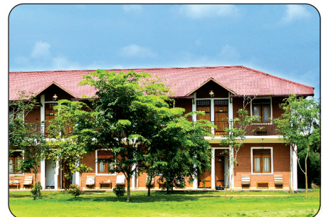
Roof & Wall Panels
