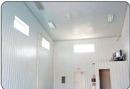
Interior Wall & Roof Liners
